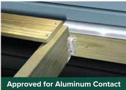
Better Corrosion Protection
